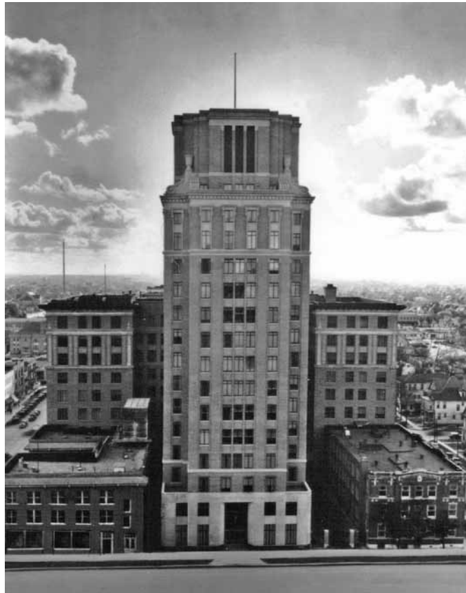
The Humble Tower, completed in 1936, was the first city building constructed with air conditioning. Architects hid the cooling tower in the penthouse.
