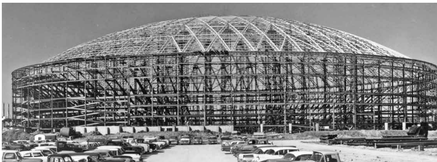
By January 1, 1964, the outline of the Astrodome was clearly visible to families who drove to the outskirts of Houston to see the steel skeleton rising on the prairie.
