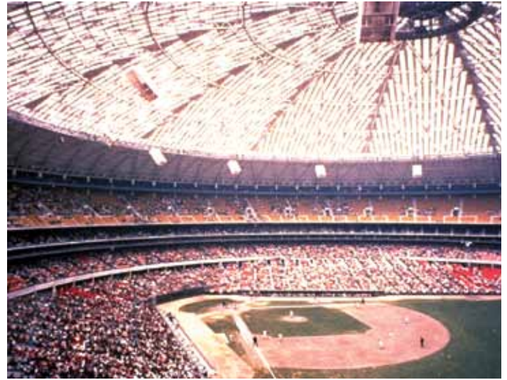
The glare during day games created a comedy of errors before the roof was painted.
