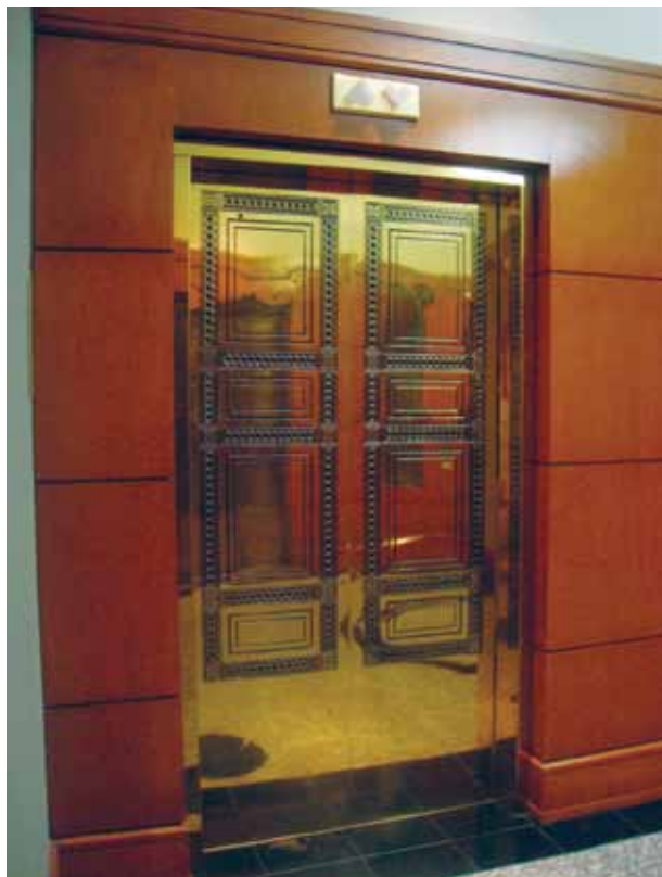
The brass elevator doors with intricate detail were refurbished to their original condition.
