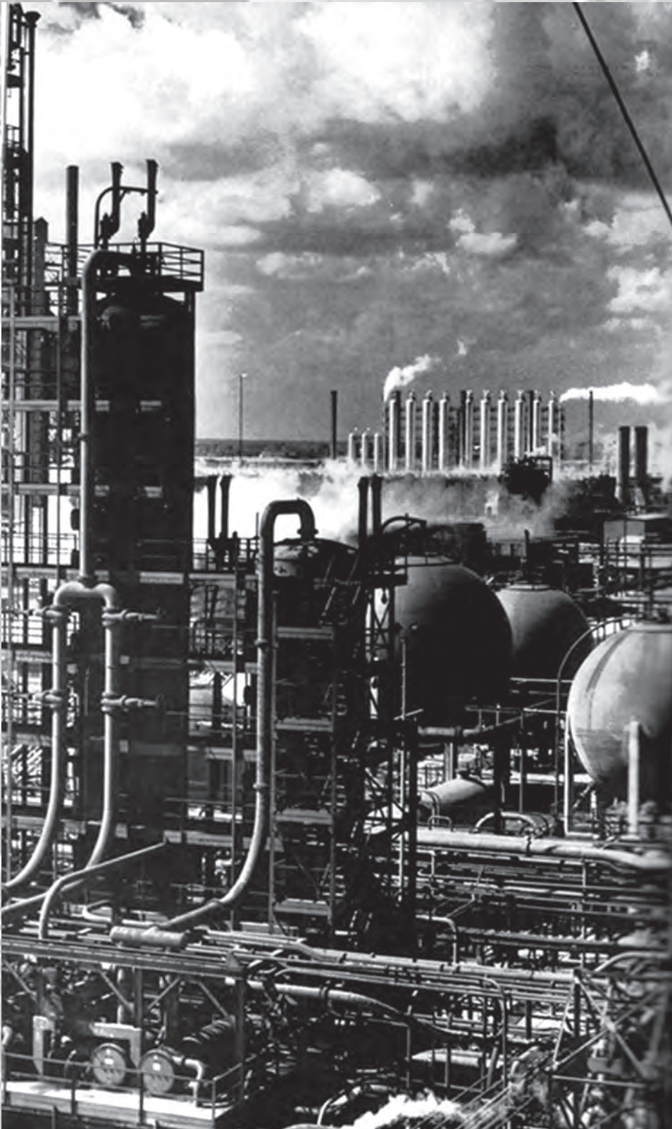
A view of the center of the Baytown refinery during World War II. The light-ends fractionating towers are in the foreground, and the toluene facilities are in the background.
