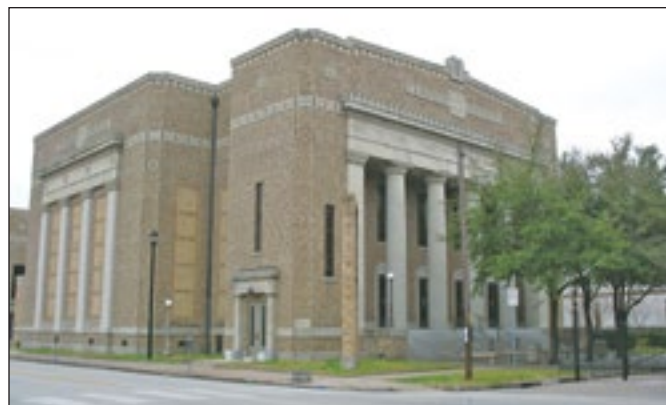
Built in 1925, Temple Beth Israel was designed for Finger’s own Jewish congregation. Beth Israel used the structure until 1967. Today it serves as the Heinen Theater of Houston Community College.
