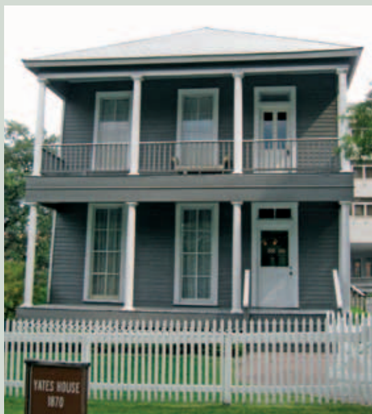
Originally built in 1870 at 1319 Andrews Street in Freedman's Town by Reverend Jack Yates, the Greek Revival structure serves as a repository of Yates family belongings. The home was moved to the park in 1994.
