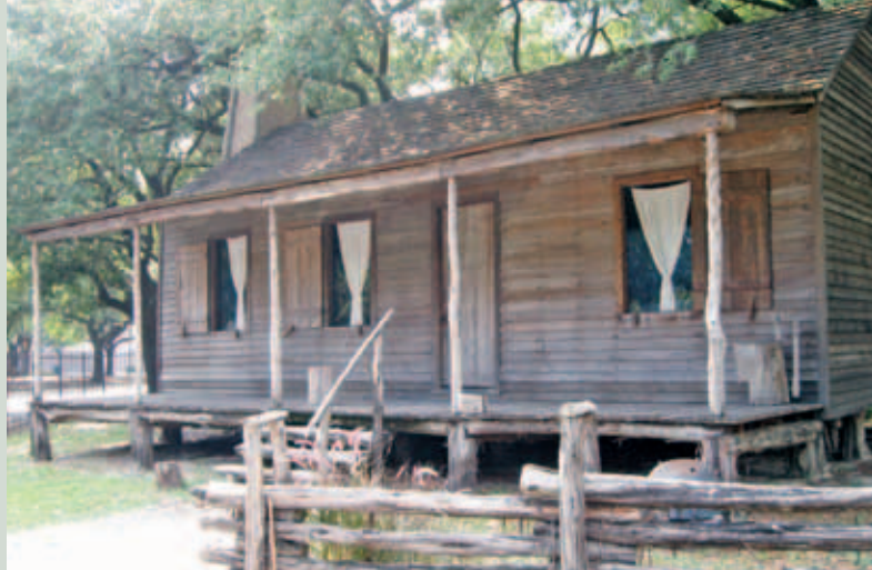
Old Place was moved from the west bank of Clear Creek to Sam Houston Park in 1973. Its roughly hewn cedar logs and mortise and tenon jointure represent defining elements of Texas frontier architecture. The cabin's interpretive features illustrate the hardships faced by early settlers.
