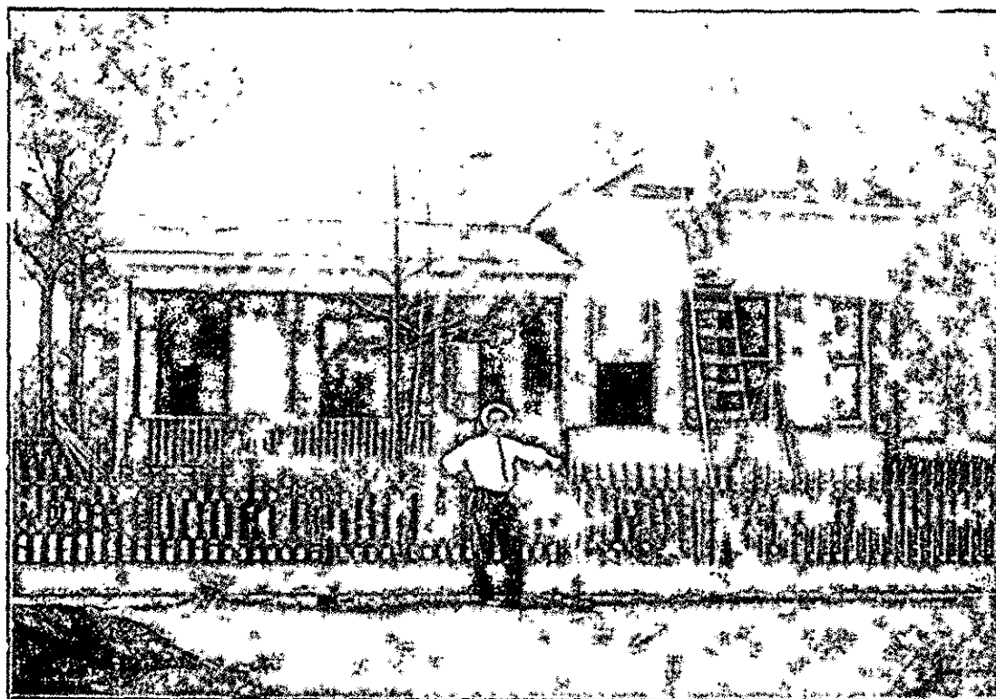
The company's advertising brochure used this photograph, apparently of a proud homeowner, to illustrate "Samples of Homes Being Erected in Magnolia Park."
