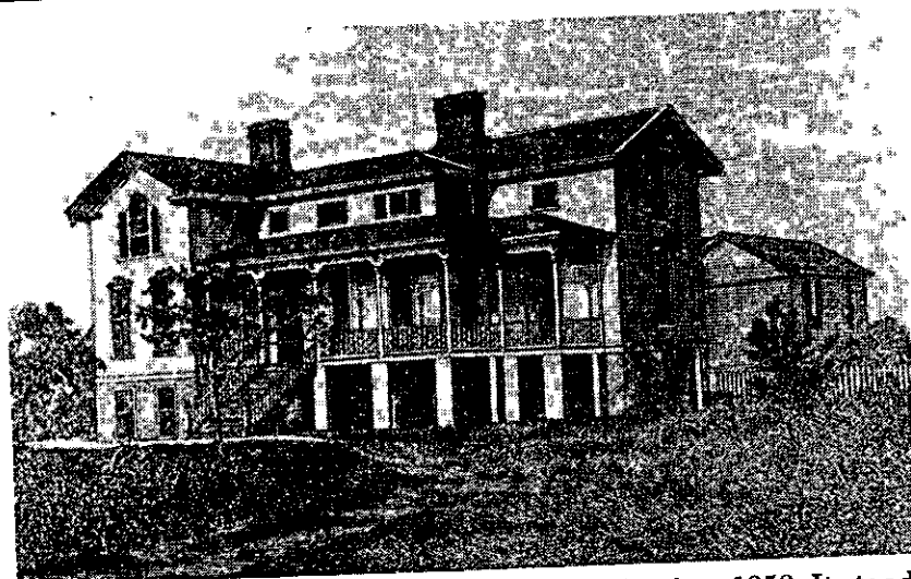
Edward H. Cushing's house, "Bohemia," was built circa 1858. It stood on a 10-acre site now bordered by Holman, Elgin, Austin, and San Jacinto streets. Cushing's garden was famous for its many exotic varieties of flowers. The land on which Forsgard later built his house was adjacent to Cushing's property.
