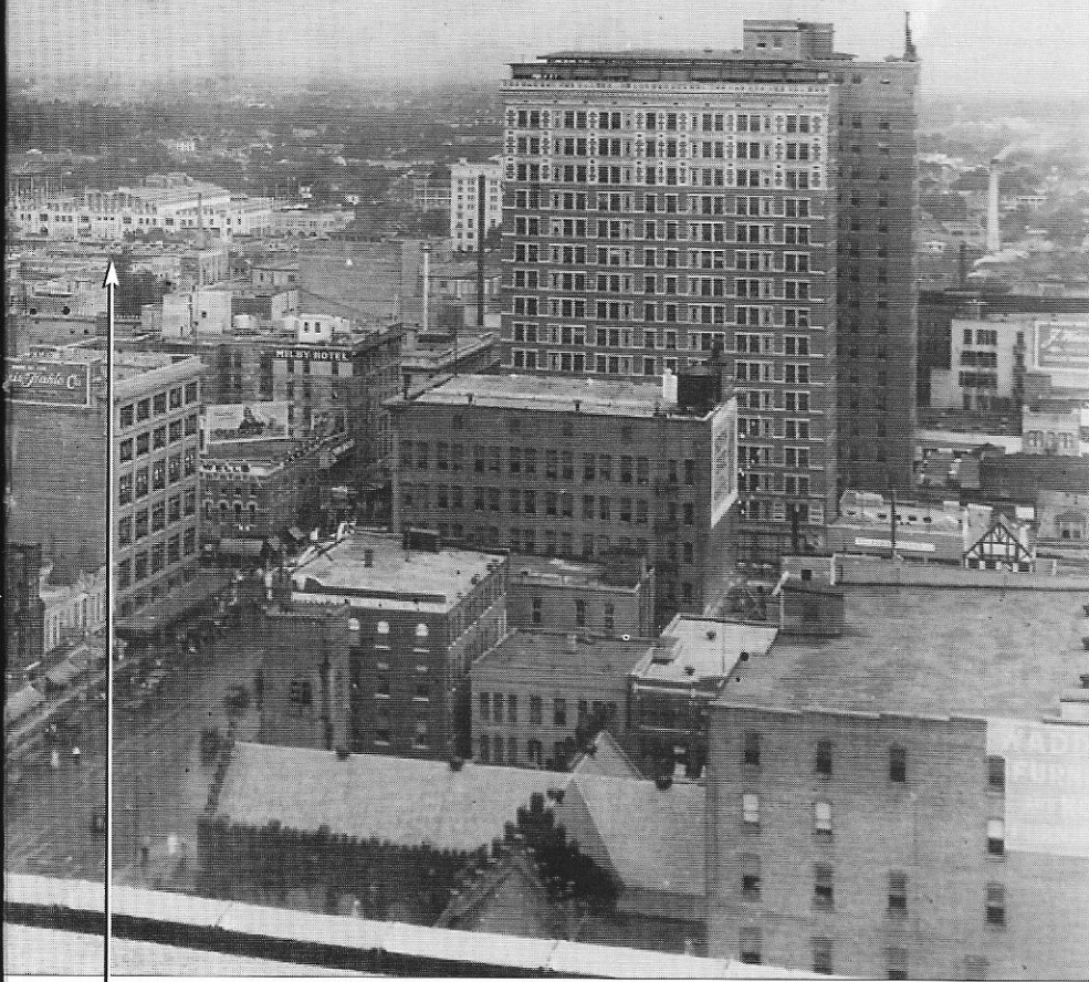
completion in the center; and the skeleton of the Gulf Building under construction on the left.
