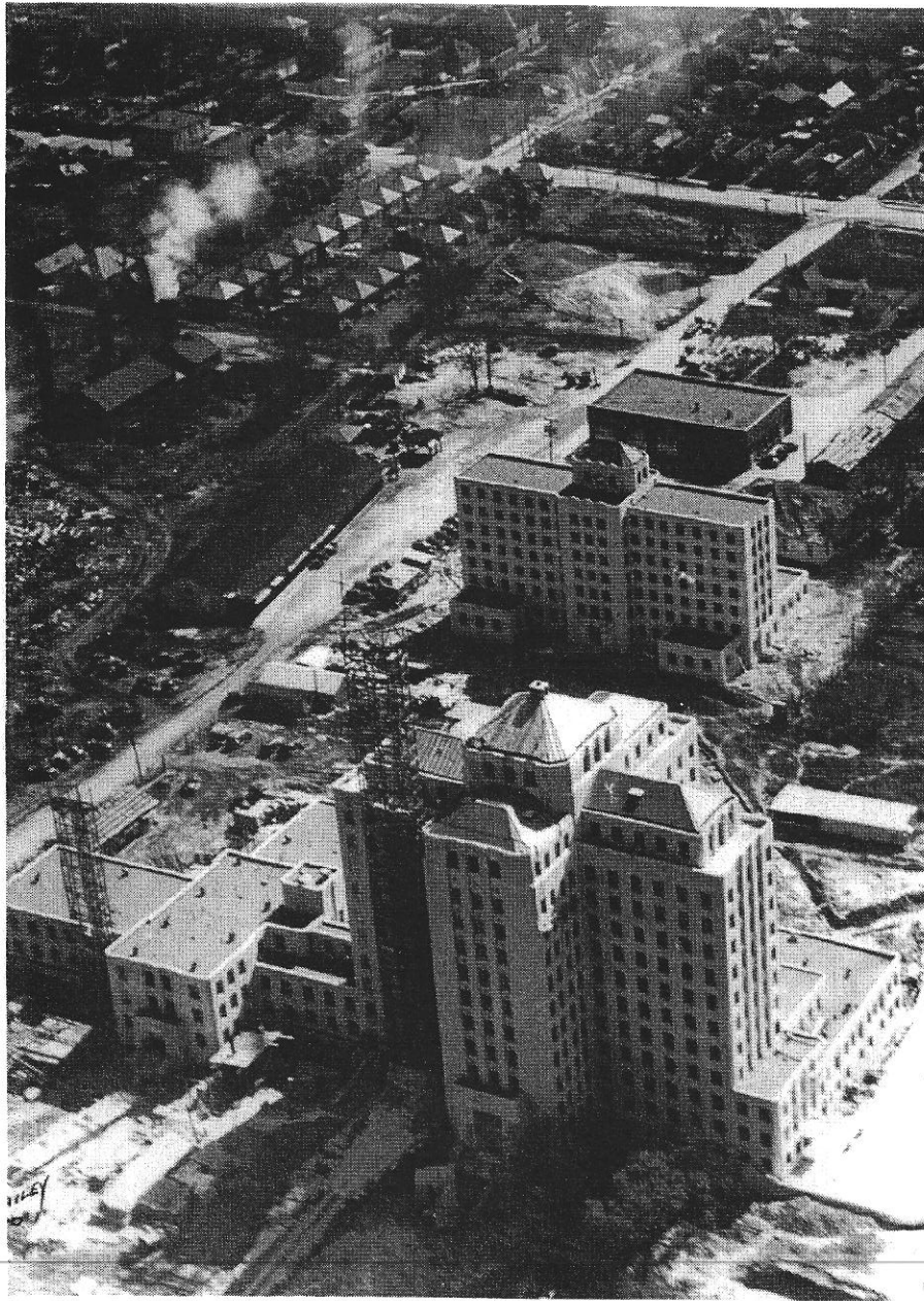
Aerial view showing Jefferson Davis Hospital and the adjacent nurses home under construction, ca. 1937. The cornerstone of the hospital was laid on July 8, 1936, and the building was completed on October 28, 1937. The hospital was located on Buffalo Drive, which was later replaced by the Allen Parkway.
