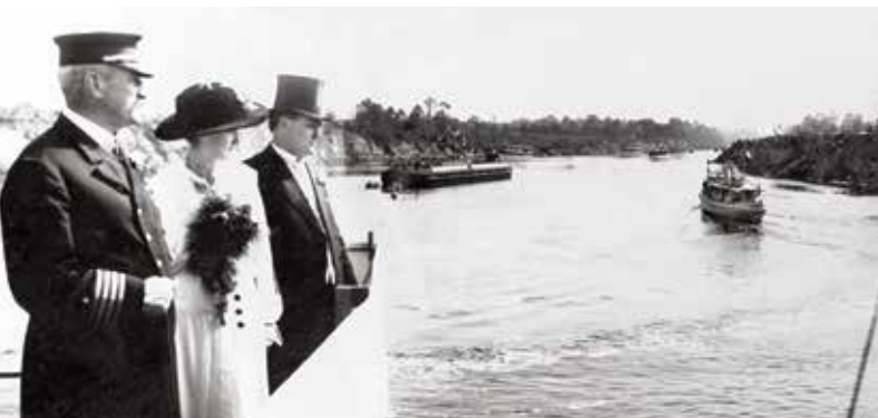
At 11:00 a.m. on November 10, 1914, the daughter of Houston’s mayor, Miss Sue Campbell dropped rose petals onto the water and christened “Port Houston.” Photo courtesy of Story Sloane Gallery.
