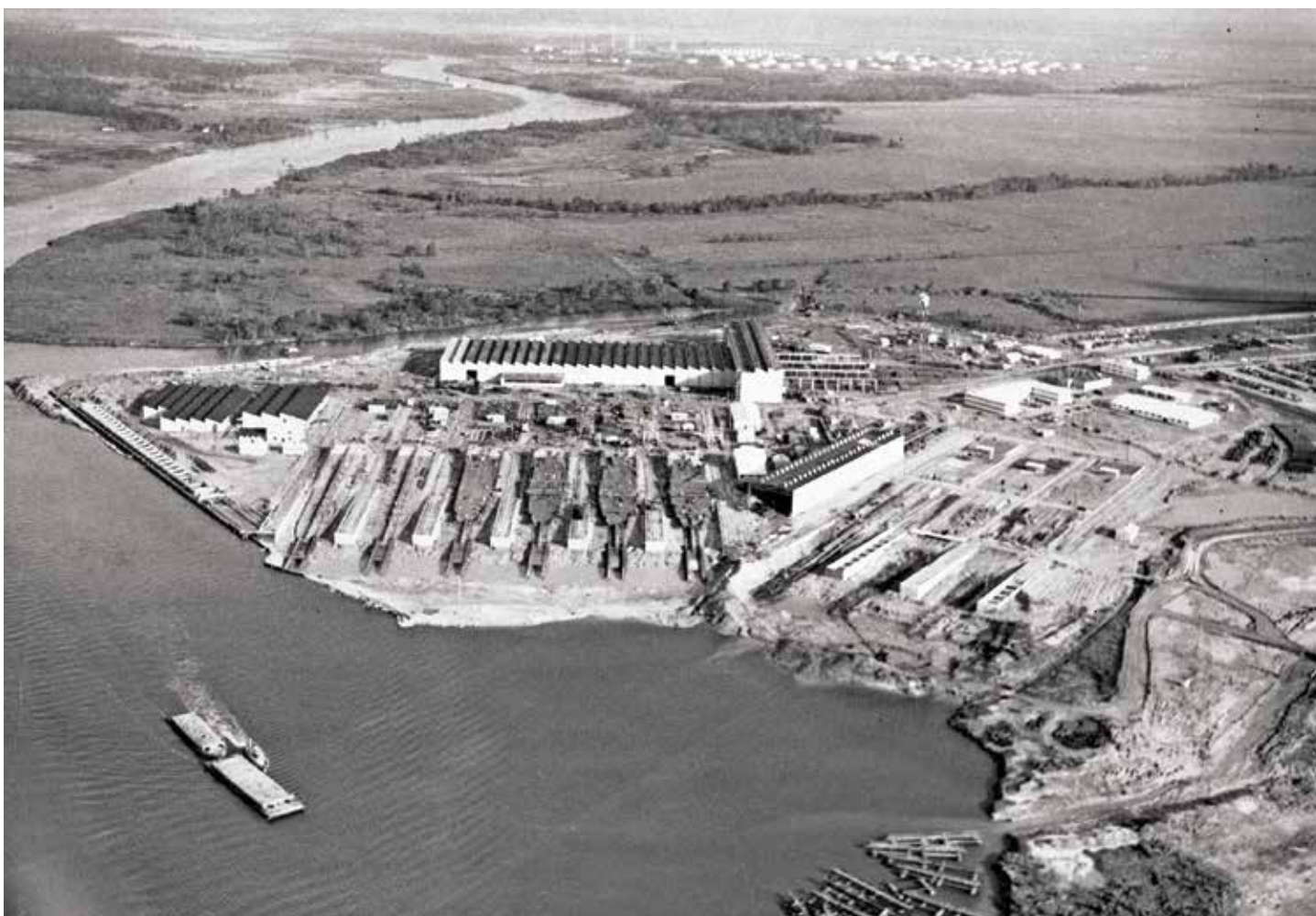
The aerial view of Houston Shipbuilding Corporation's shipyard in 1941 shows the first four Liberty ships under construction (center). The ends of the building slips had not yet been dredged for launching.
