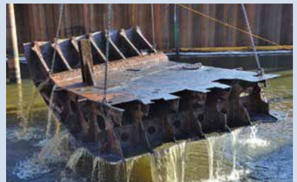
Lifting out a section of Davy Crockett’s double bottom, August 18, 2011.
