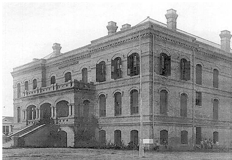
This postcard shows the Galveston Orphans Home in the early 1900s, following repairs made in the aftermath of the 1900 Storm.
