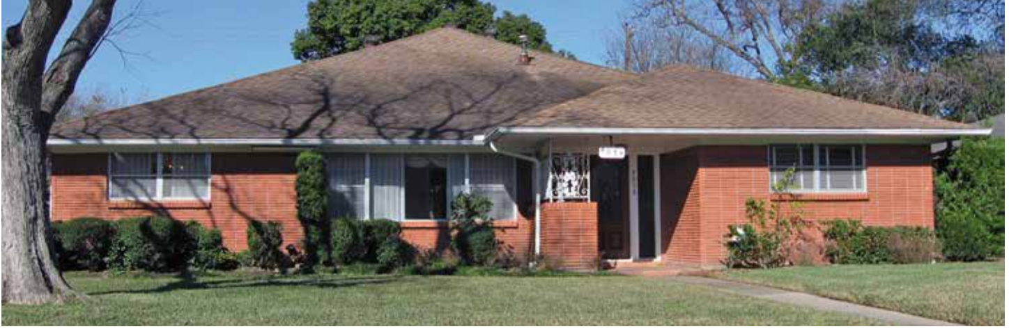
Builders simplified and mass-produced the ranch house in the 1950s. Also called a tract house or a rambler, this example has the popular hip roof with wide eaves and a prominent picture window. Photo courtesy of the author.
