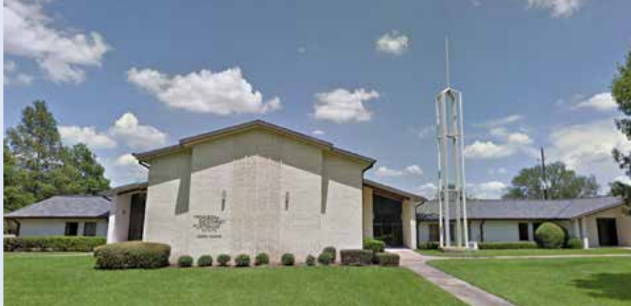
Church members built the Drexel Building from the ground up.
