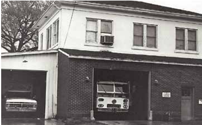
Some fire stations had to add on to accommodate an ambulance.
