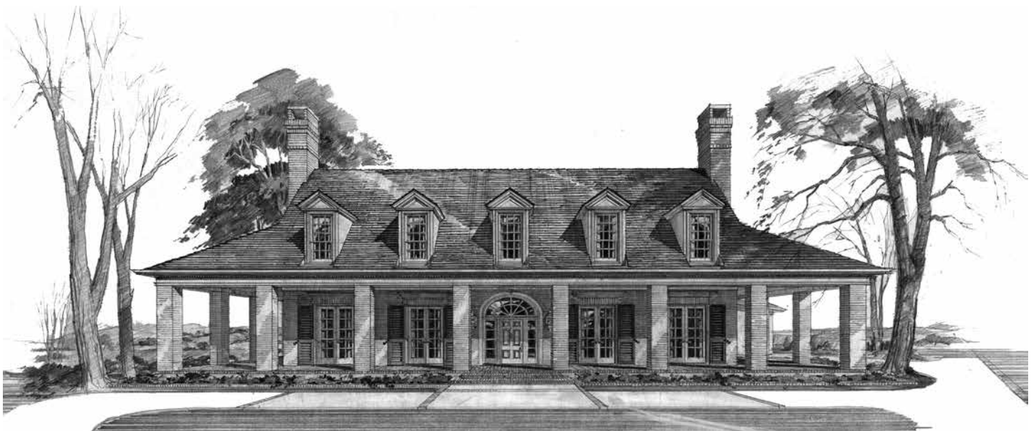
Lucian T. Hood, Jr., 4307 Churchill Downs Drive, Austin (1983). Hood interpreted Texas regionalist precedents for this Hill-Country commission but executed the house in a buff-colored brick rather than native limestone. The design was specific to its site and departed from the Georgian Revival and French Country styles that characterized most of Hood's houses in the Houston area during the 1980s.
