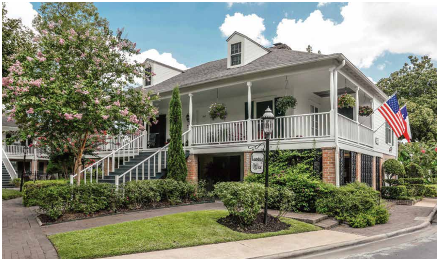
Lucian T. Hood, Jr., Memorial Creole Apartments , 10220 Memorial Drive, Houston (1968).
