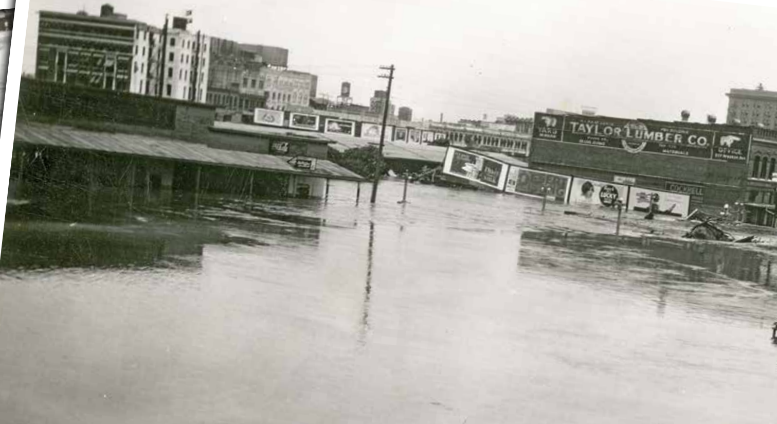
Looking north toward the Southern Pacific Station from the Preston Avenue Bridge, flood waters lap at the bottom of billboards. RGA21a-021.
