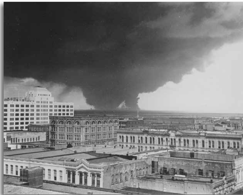
The cloud of smoke in this photograph, taken from a Galveston rooftop, explains why many descriptions compared the Grandcamp explosion to that of an atomic bomb.
