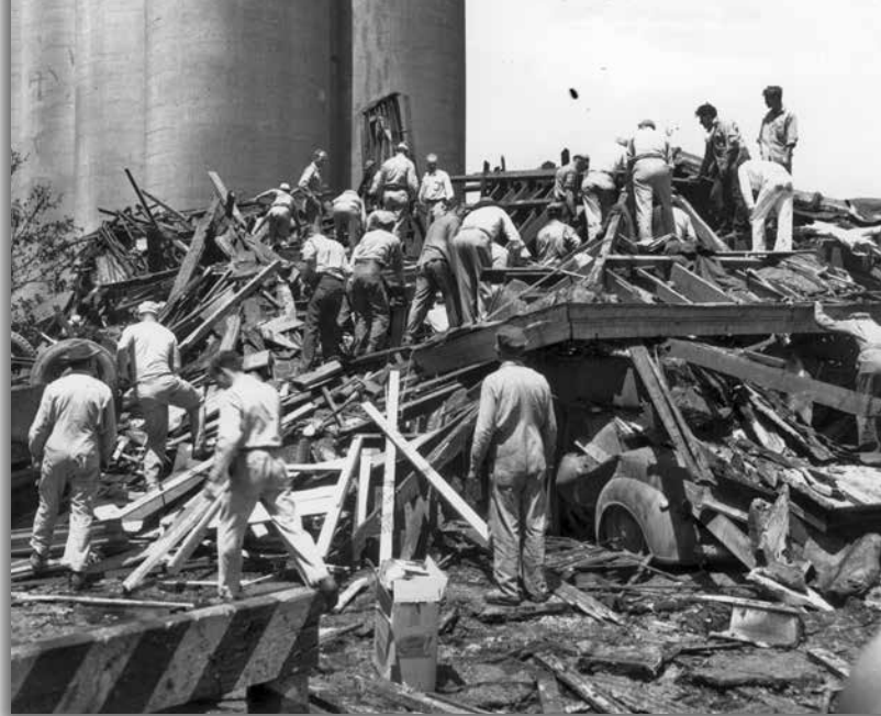
Alongside a grain elevator, rescue and recovery crews search through a pile of metal girders, a collapsed roof, overturned and crushed cars, and other debris measuring nearly ten-feet high.
