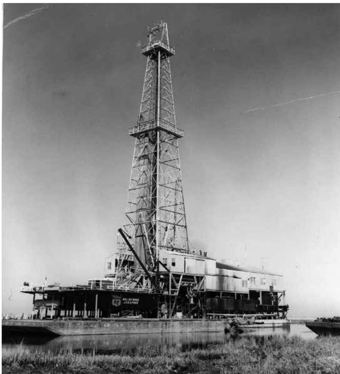
*Drilling barge used for marsh and shallow bay drilling to develop networks of canals in coastal Louisiana, circa 1960.*
