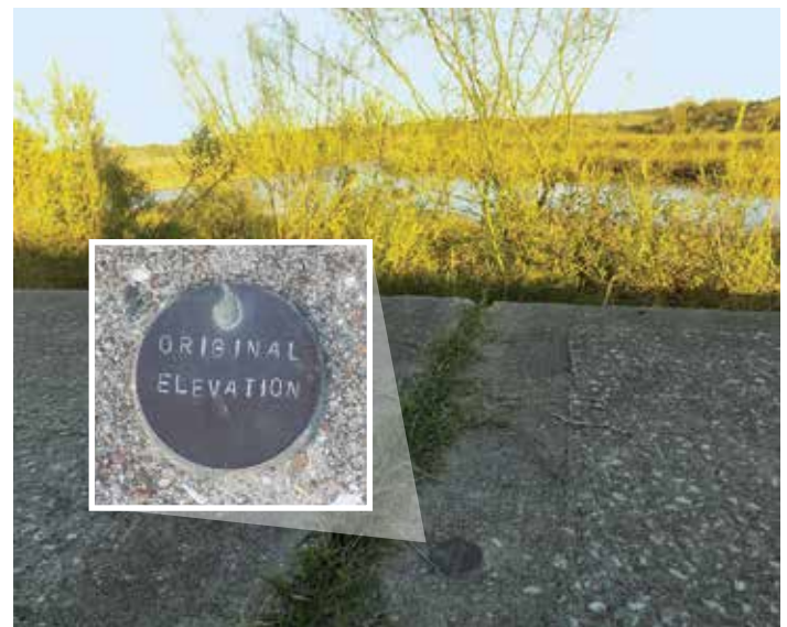
The City of Baytown installed this medallion at the Brownwood Educational Pavilion to indicate the peninsula’s original elevation in comparison to the vegetation and water in the background, which are noticeably lower due to subsidence.
