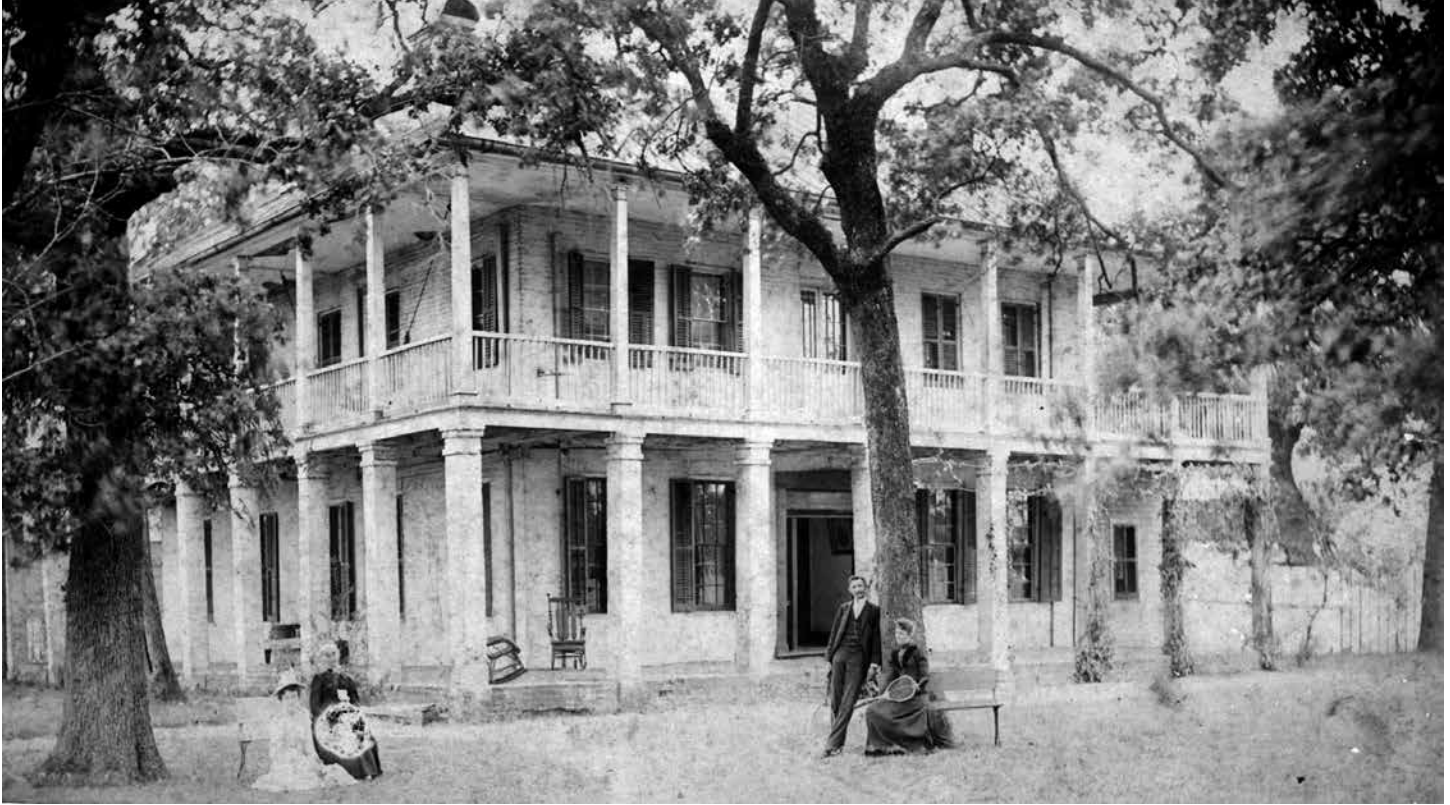
The Noble family in front of their home, circa 1890. Two features differ significantly from the house's twentieth-century appearance: The roof is clad in standing seam metal with a half-round gutter, and the columns are more numerous and configured differently than today. Closer inspection reveals a slightly different balustrade and a different pair of doors on the primary façade upstairs.
