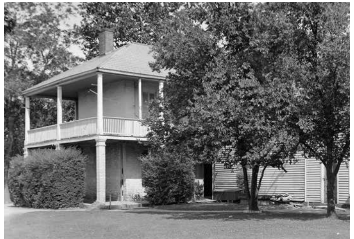
This photograph, showing the enclosed balcony on the back of the house, and its architectural drawing were part of the Historic American Buildings Survey from 1936. During the time the Kellum-Noble House (called the "Shelter House") was surveyed, it served as the Parks Department headquarters.
