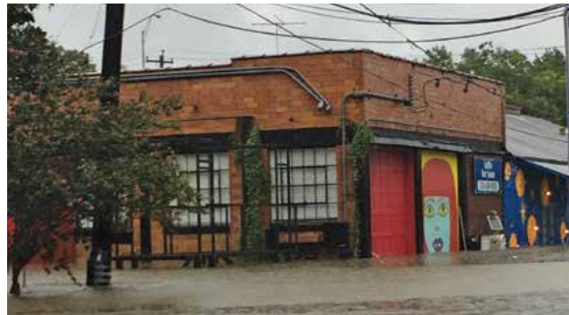
Water rose around Wayne Wilden's hundred-year-old warehouse, now converted to apartments, during Hurricane Harvey. The stairs leading up to the Starry Night-inspired façade are completely submerged.
