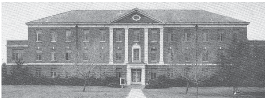
Designed by PVAMU alumnus Louis Fry, the third iteration hospital, along with other buildings at this time, were constructed using solid brick to prevent fires like the one that brought the second iteration hospital to its demise.
