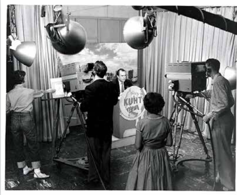
UH raced to expand the KUHF radio facilities to accommodate a television broadcast studio. It also conducted nation-wide searches for staff with television broadcast expertise who could grow the radio communications program to include television.
